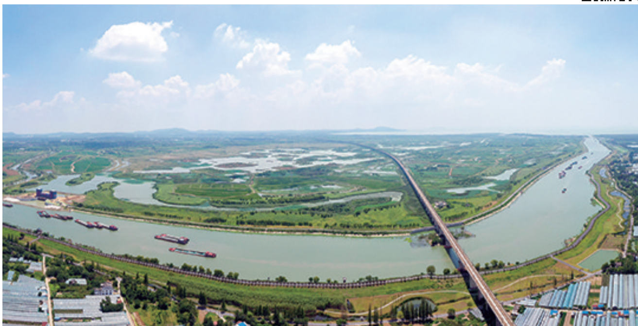
十八联圩生态湿地蓄洪区俯瞰
